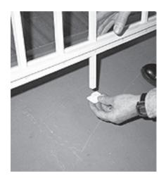
**Note:** If you are installing the Railing on a concrete patio, you will have to mark the location in the same manner as above. Use a 1/4" masonry drill bit and drill 1-1/4" deep. Install a plastic lag shield and install the #10 x 1" hex head screw in the same manner as above.
