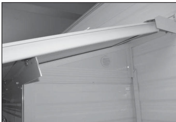
After Gable End
