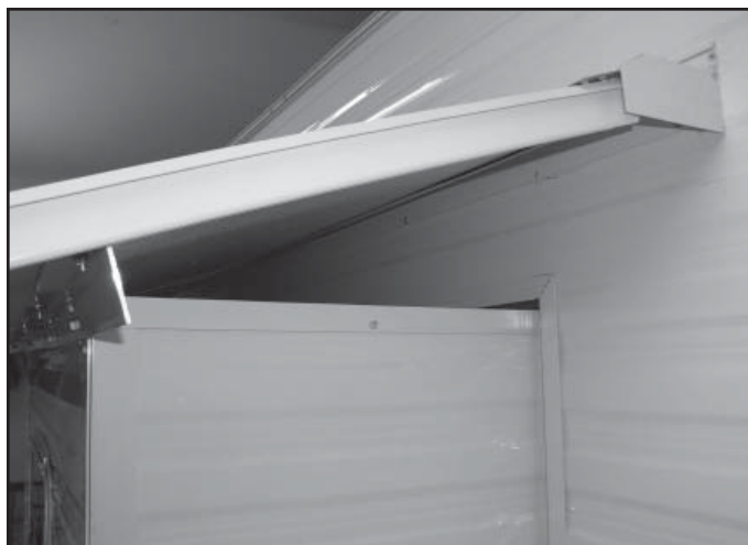
Before Gable End
