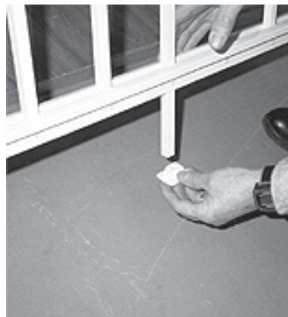
**Note:** If you are installing the Railing on a concrete patio, you will have to mark the location in the same manner as above. Use a 1/4" masonry drill bit and drill 1-1/4" deep. Install a plastic lag shield and install the #10 x 1" hex head screw in the same manner as above.
