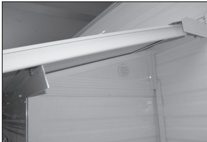
After Gable End
