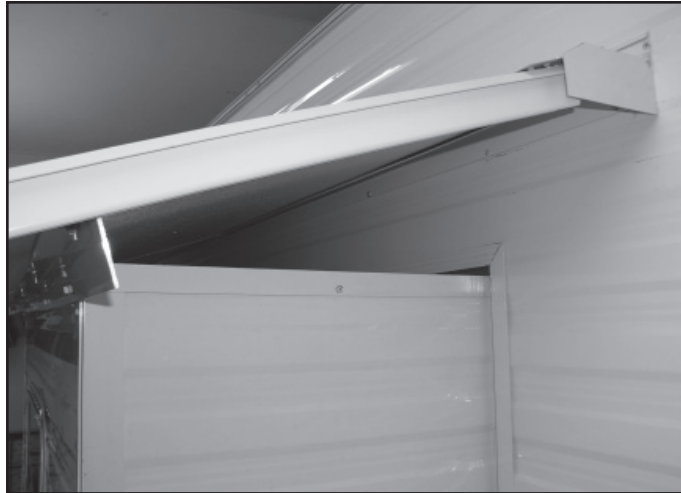
Before Gable End
